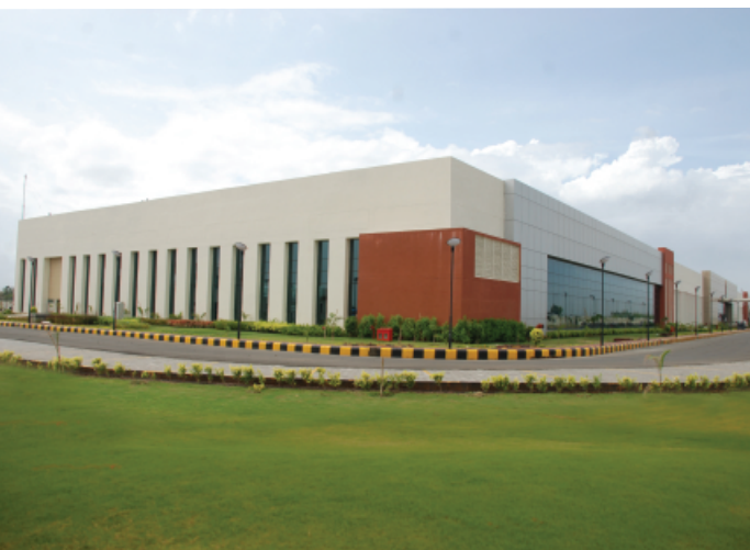
Switchgear Factory, Baroda
